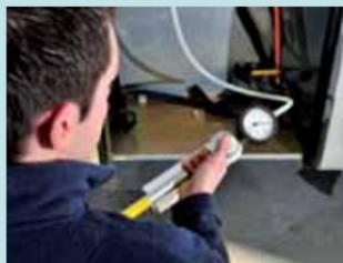
Lee (pictured here) went around the outside of the 'van and inspected the gas lines, testing the pressures: if they dropped, it would indicate a leak somewhere in the system.
