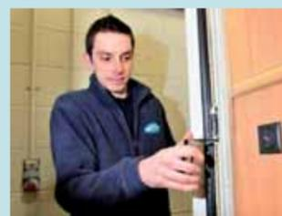
When he checked the doors, Lee found a gap that was slightly too wide and causing a problem with a catch. He adjusted it by moving the hinge across slightly, allowing it to sit better in the frame.
