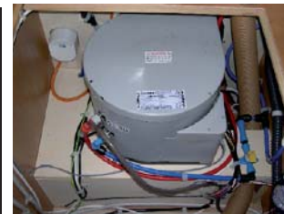
The boiler supplies hot water, and so is a vital part of the system
