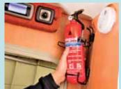
The fire extinguisher was taken from its mounting to make sure it was free, and fully charged, just in case it is ever needed. (An important check for us all. See G. O'Neill's letter on page 29)
