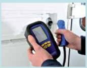
After checking their seals for cracks. Lee made sure that the flues were working. He used a probe to check the system emissions to ensure that there was no carbon monoxide, and that the flue was not blocked.
