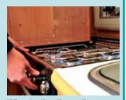
When testing the appliances, the main check was on the gasburning hob. Lee made sure the flames were blue, and did not turn yellow, or flare, which would be a sign of a blocked flue or stove plate, resulting in the release of carbon monoxide.
